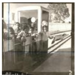
Khel Gaon Station at Bal Bhavan, 1959. (Khelgaon9_06 Dec 1959)
