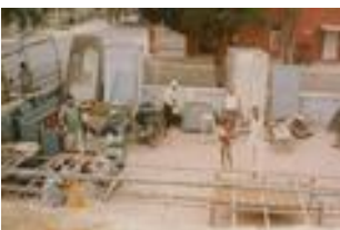
Nirankari Bhavan undergoing construction (ST- 24)
