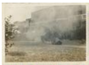
Building clouded in smoke during the Air Raid Precaution drill. (LNP-B-025iii)
