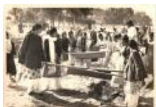
Students participating in swimming pool construction work, 1940. (IP_021)
