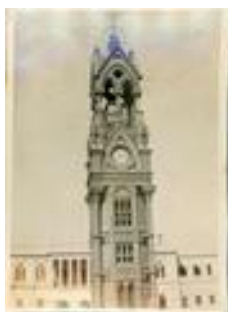
Ghantaghar or the Northbrook Clock Tower, Old Delhi (LNPIII_052)
