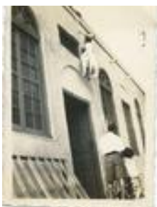
Evacuating by knotted rope-ladder. (LNP-B-025vii)
