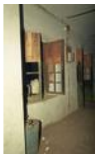
A corridor at Anglo Sanskrit Victoria Jubilee Sr. Sc. School (LNPIII_SC017)
