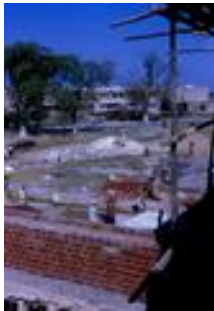
Construction at Okhla Marg (JF_0005)
