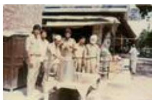
Early construction of Sant Nirankari Satsang Bhavan in Nizamuddin (ST- 01)
