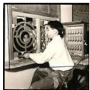
Khel Gaon Station at Bal Bhavan. (Khelgaon11_06 Dec 1959)
