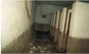
Wahsrooms at Anglo Sanskrit Victoria Jubilee Sr. Sc. School (LNPIII_SC031)
