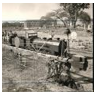
Khel Gaon Station at Bal Bhavan. (Khelgaon8_06 Dec 1959)
