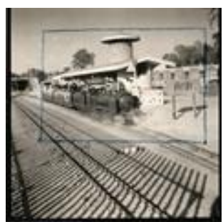
Khel Gaon Station at Bal Bhavan. (Khelgaon10_06 Dec 1959)
